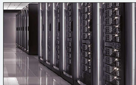
Power Distribution Units
