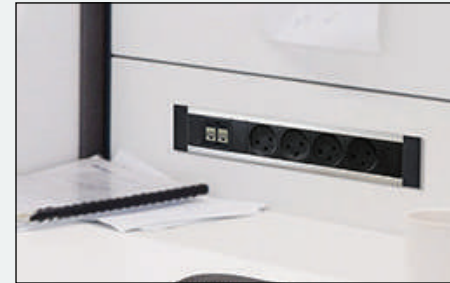
In the barrier / panel
